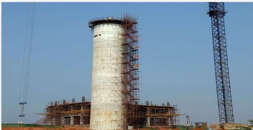
Airport will have state of the art ATC tower with modern facilities and equipments. The ATC centrally located towards west of the terminal building, is provided with a ground level entrance, tower level 1 will be technical, tower
