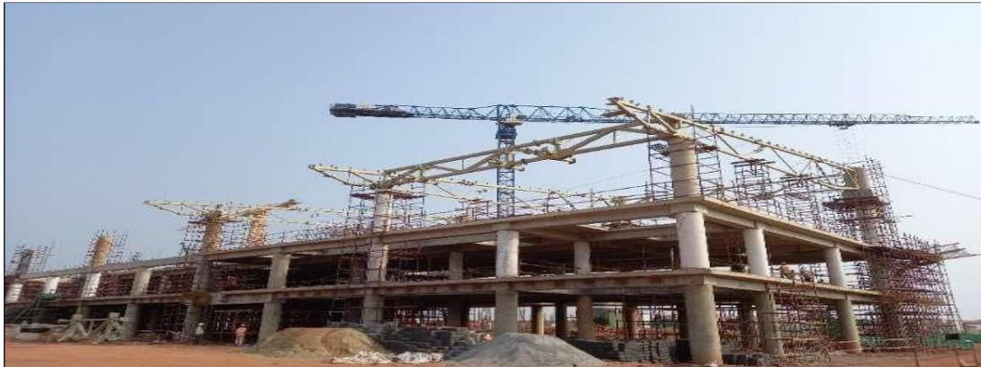
The Integrated Passenger Terminal Building has design capacity of 4.4 mppa in phase I following by 5.8 mppa, 9.4 mppa and 13.1 mppa in phase II, phase III and phase IV respectively. It will be a three level terminal building where ground level or apron level is for departure & arrival of aircraft parked at remote base, Level 1 is for arrivals through boarding bridges and Level 2 is for departures through
